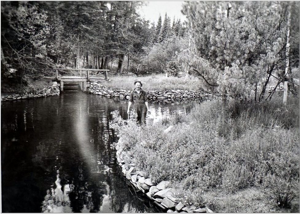
Herman Turpa, the station’s caretaker, with his feeding bucket in the stone-lined race — July 1935. (Photo: A.L. Wilson, Fish Division)
