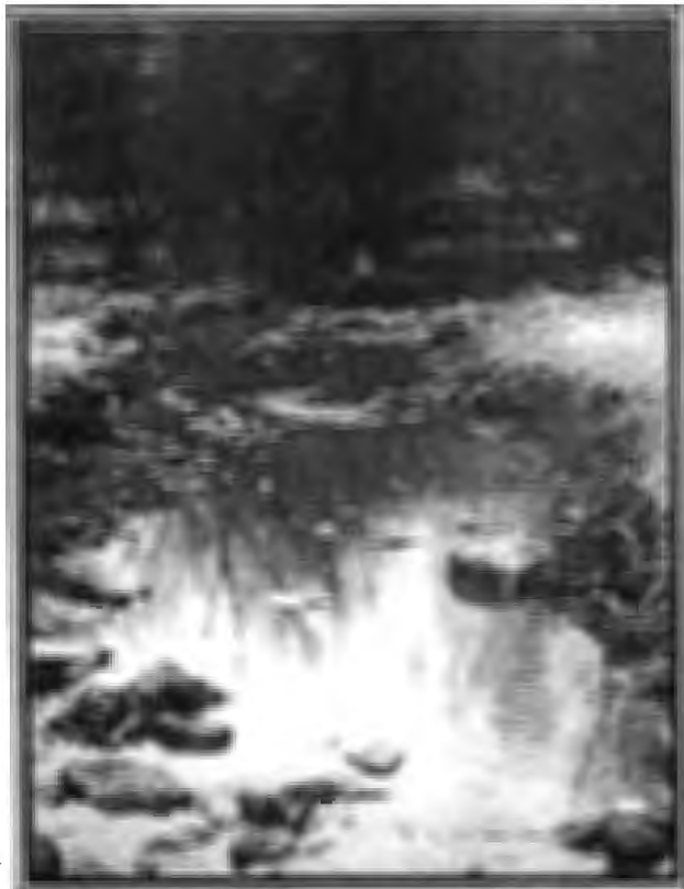
Below: Middle section of storm drain, facing the Iron River. The vegetation in the foreground of the basin has encroached over previously accumulated sediment and is representative of what the entire basin looked like prior to maintenance. Notice the new plume of sediment beginning on the right side of the channel.
