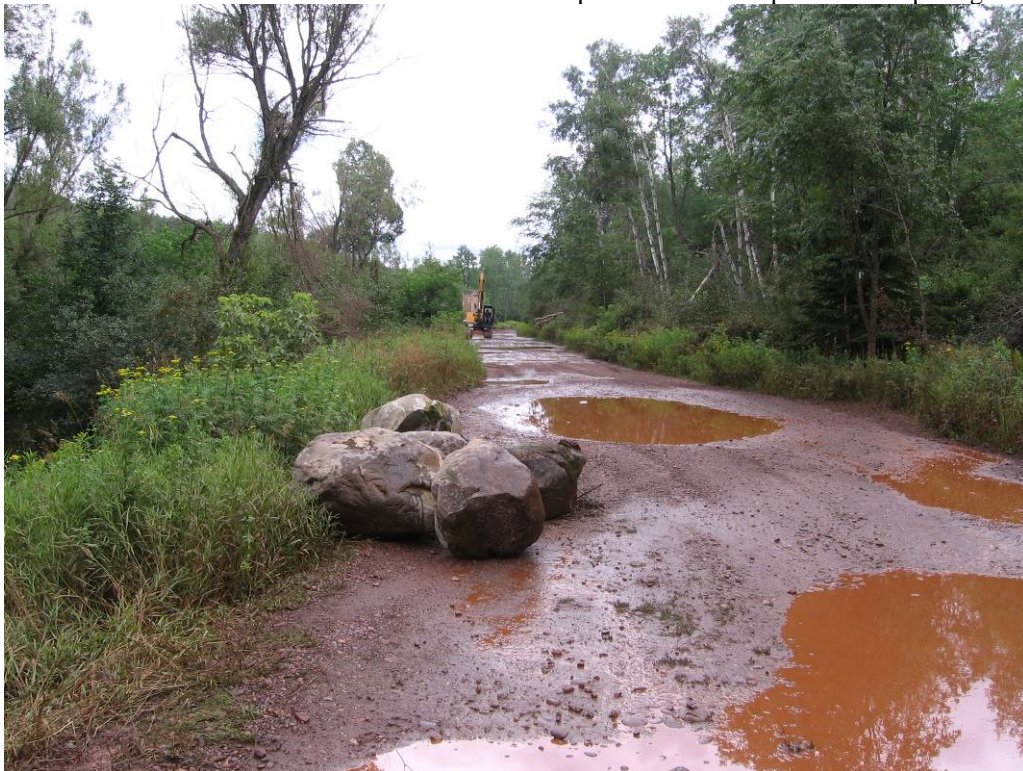
Figure 45: Runoff from the ORV trail contributes suspended sediment to the adjacent river
