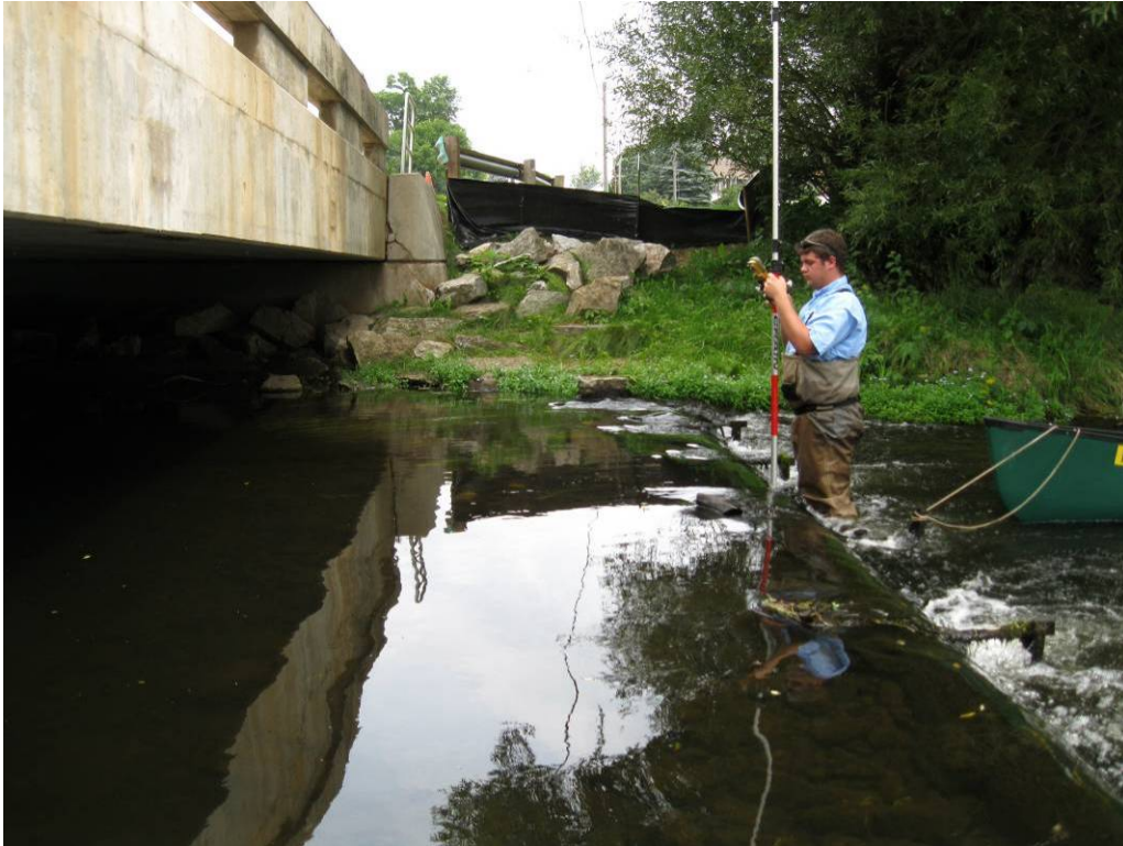
Figure 38: Sewer or stormwater pipe crossing at 4th Ave. This crossing is a fish barrier and should be retrofitted or removed to accommodate fish.
