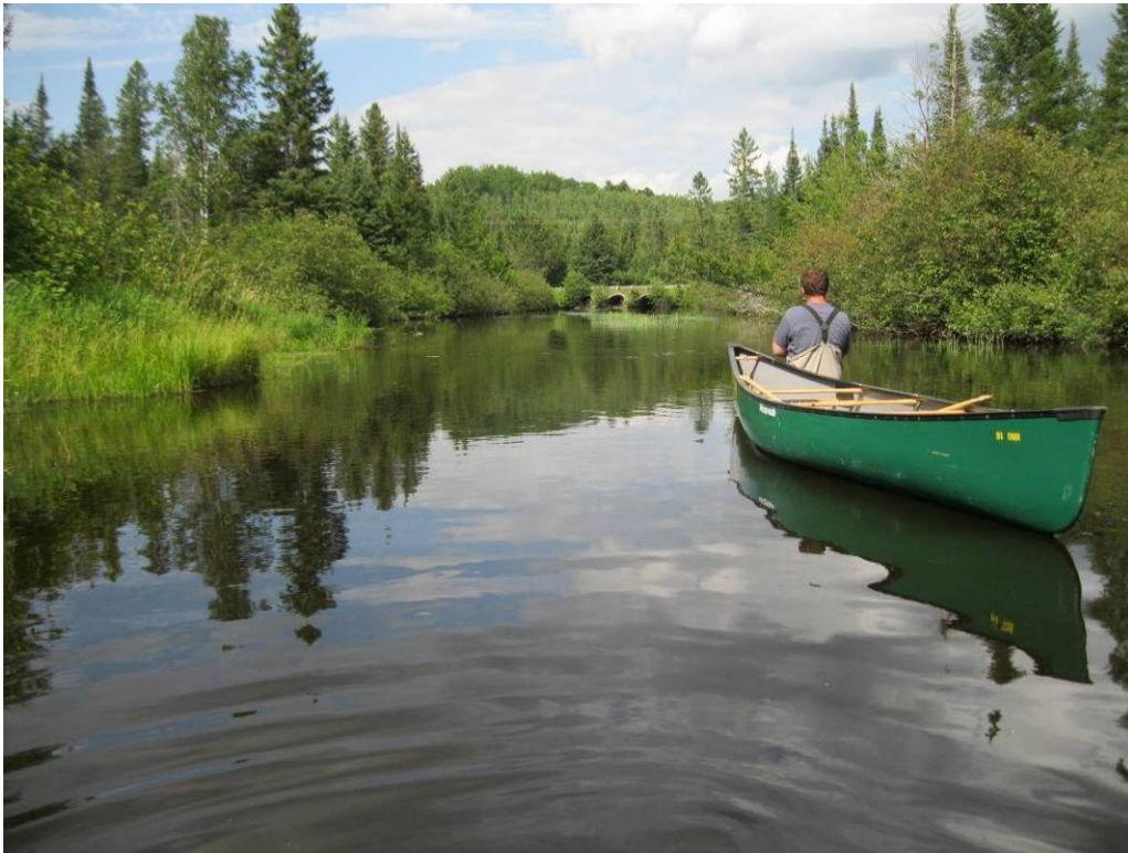
Figure 24: Three culverts at Gibbs City Rd. Note the slack water and presence of aquatic vegetation occupying sediment deposits in the channel.
