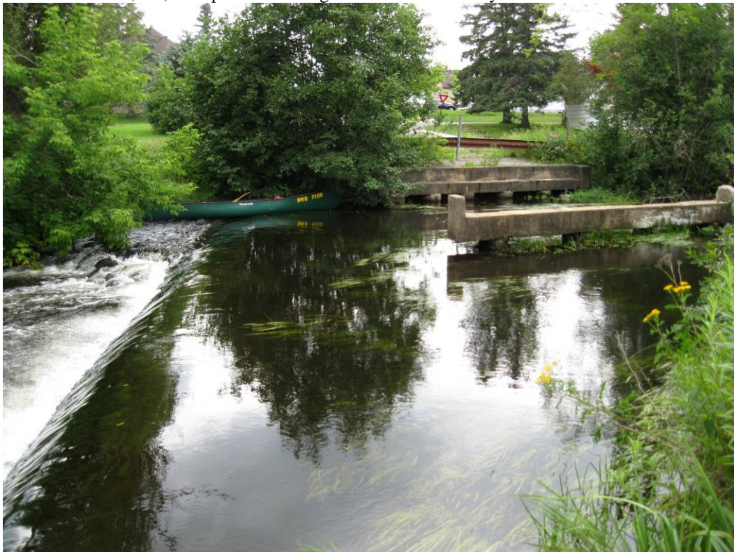
Figure 37: The dam at 5th Ave. A fish passage barrier it should be removed and if necessary replaced with a riffle.
